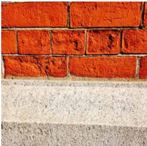
1. Red brick with lime mortar and English bond
