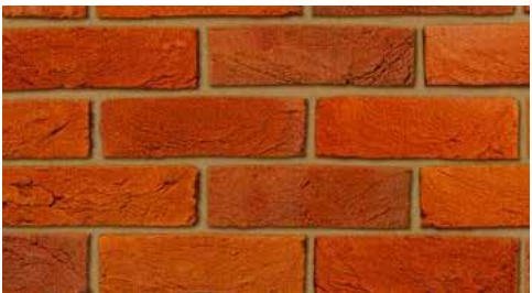
1. Swanage multi-red brick, English bond (not shown) and lime mortar
