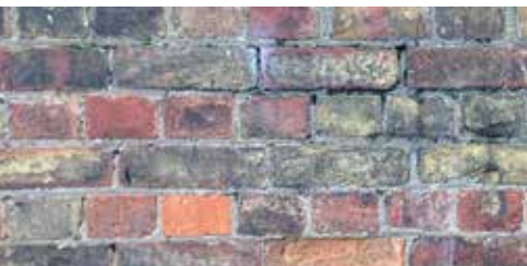
3. Range of weathered bricks, lime mortar and English bond
