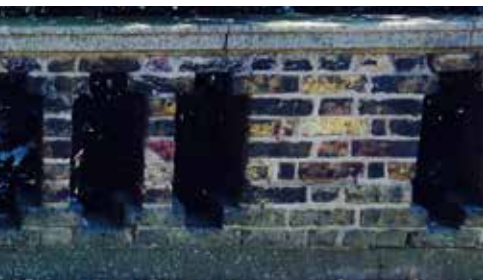
4. Brick and concrete capping decorative wall
